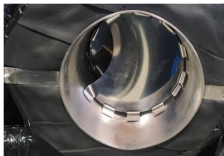
Fig. 3. Vapour trap with opened lid
